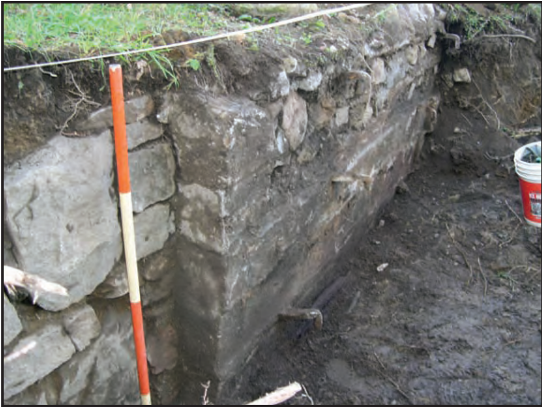
Plate 27. View looking southwest of the south wall of the lock in Trench 1 showing the mortar repairs poured behind the locks missing timber sheeting; note the horizontal timber sheeting visible along the wall at the base of excavation (Photographer: James Lee, October 2006) [HRI Neg.#06052:D3:14].
