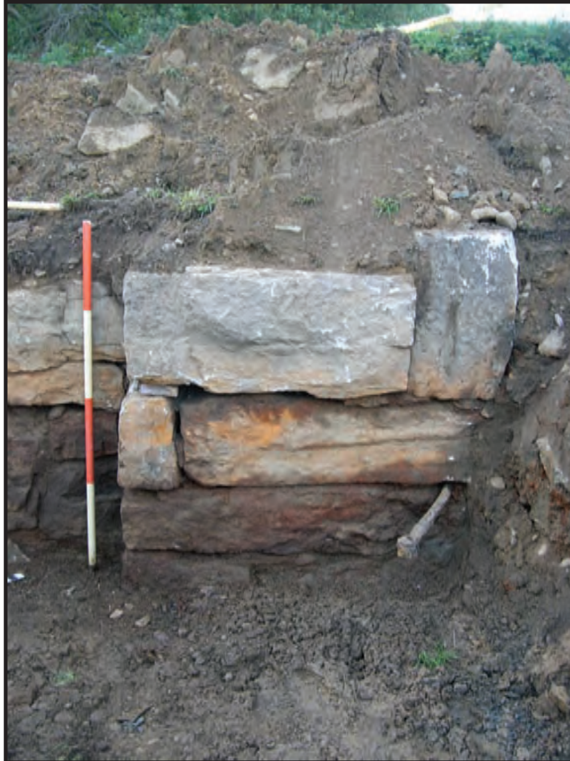
Plate 32. View south of the south wall of the lock showing an iron tie-rod that probably held timber bumpers used to guide the boat into the lock (Photographer: James Lee, October 2006) [HRI Neg.#06052/D3:33].
