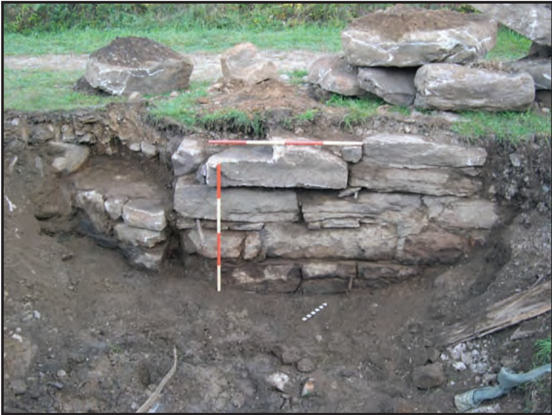
Plate 33. View looking north of the north wall of the lock exposed in Trench 2. The flaired, upstream headwall of the lock is visible at the left end of this section. Unlike the wall opposite this one (Plate 30), there is no recess to accommodate the drop gate mechanism, which is only necessary on one side. Also, the original top of this wall was removed when the lock was dismantled. The large flat coping stones which had run along the top of this wall were found in the lock and are visible lying on the ground above this wall (Photographer: James Lee, October 2006) [HRI Neg.#06052/D3:24].
