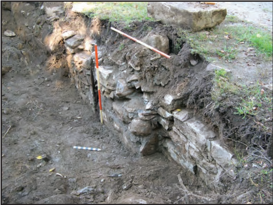
Plate 24. View northwest of the north wall of the lock in Trench 1. The recess for the miter gate is visible in the foreground and the surviving vertical timber from Plate 26 is visible next to the upright scale rod. Approximately three to four feet of the top of this wall was removed when the lock was dismantled (Photographer: James Lee, October 2006) [HRI Neg.#06052/D3:11].
