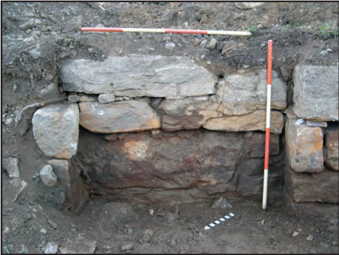
Plate 31. View south of the recess in the south wall of lock to accommodate the lever for the drop gate that was located just below the bottom of this trench (now below the water line) (Photographer: James Lee, October 2006) [HRI Neg.#06052/D3:31].
