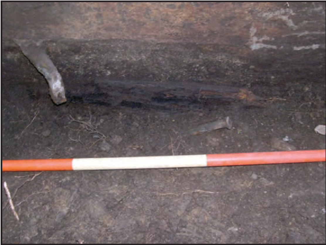
Plate 26. View south along the bottom edge of the trench against the south wall of the lock in Trench 1. A surviving horizontal timber with concrete poured behind it. The large, square spikes held the timber sheeting to the lock walls (Photographer: James Lee, October 2006) [HRI Neg.#06052/D3:15].
